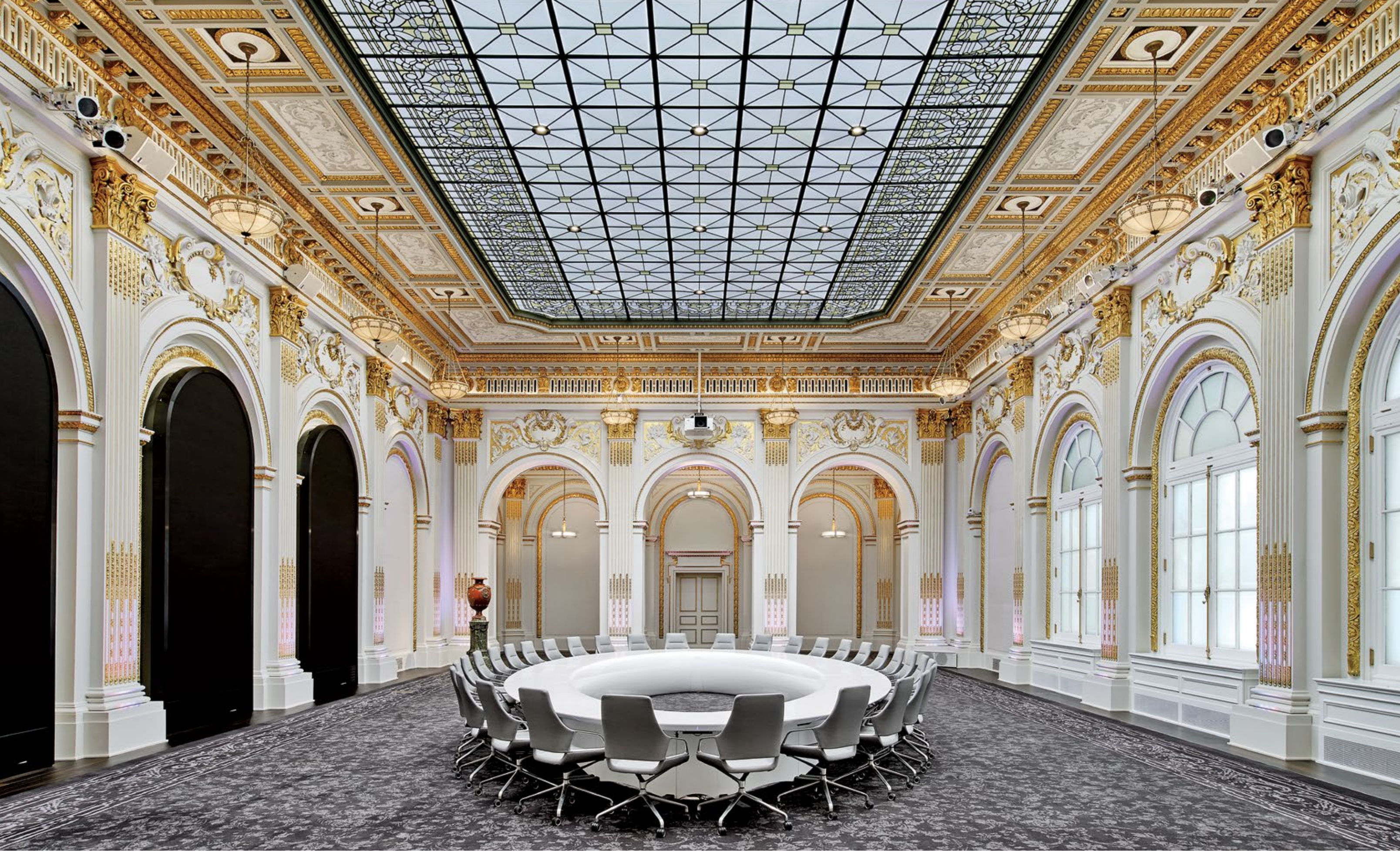
The boardroom's glass ceiling, covered since 1920, was exposed and restored, and the walled-off antechambers on either end of the room were reconnected.
