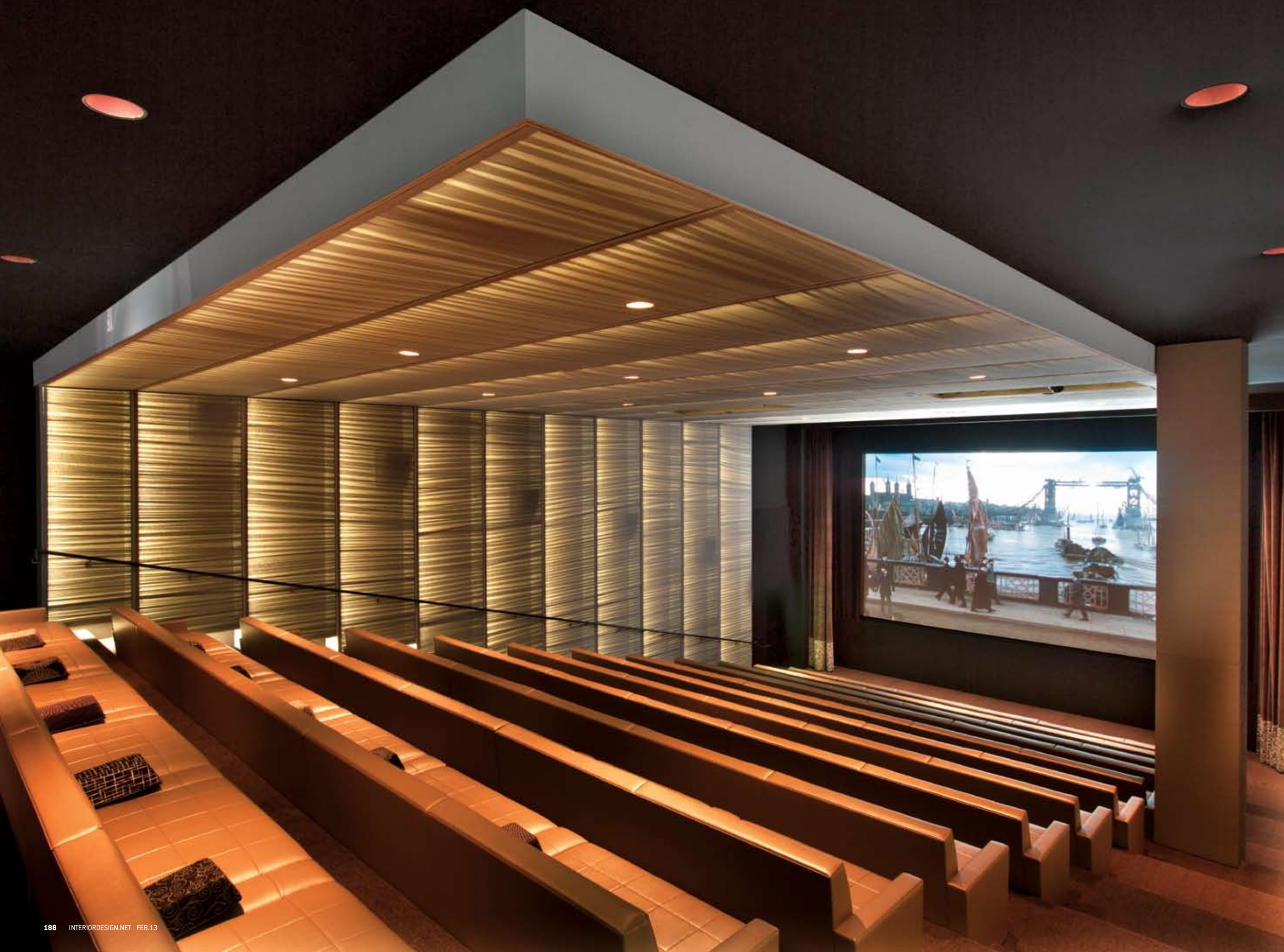
Seating 165, the screening room's custom vinyl-upholstered banquettes stand under a canopy of polyester panels.
